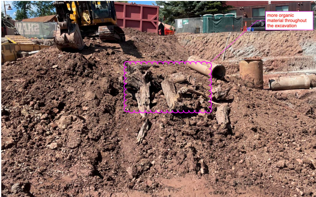
Excavation Photo 3 – Backfill Debris
