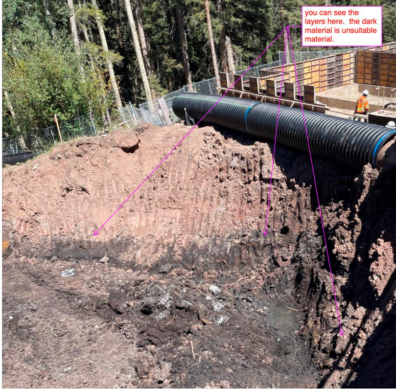
Excavation Photo 2 – Southeast Side of Excavation Adjacent to New East Building
