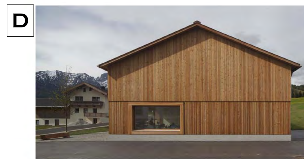
D VERTICAL WOOD SIDING
