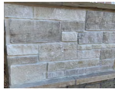
STONE VENEER: TELLURIDE STONE HERITAGE SERIES PILATUS FULL STONE VENEER
