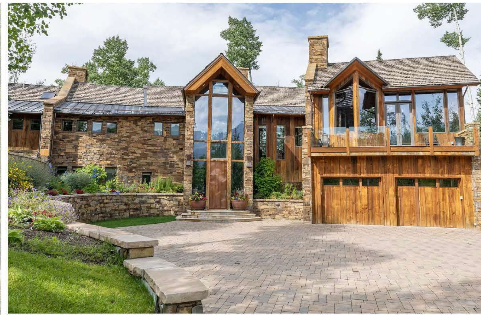
EXISTING EAST VIEW
