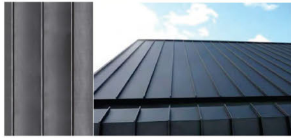
A STANDING SEAM ROOFING
