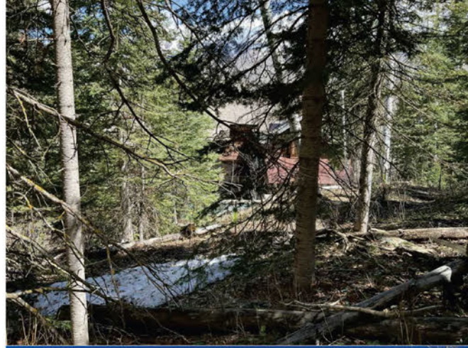
ENTRY STAIR LOOKING NORTH
